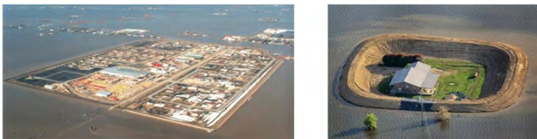
Figure 9 — Protection of an area by building embankments, levees or dykes: ring dyke at Red River, Canada (left); a levee protects a home surrounded by floodwater from the Yazoo River near Vicksburg, Mississippi, USA (Manitoba Floodway Authority, left; Getty images, right)
